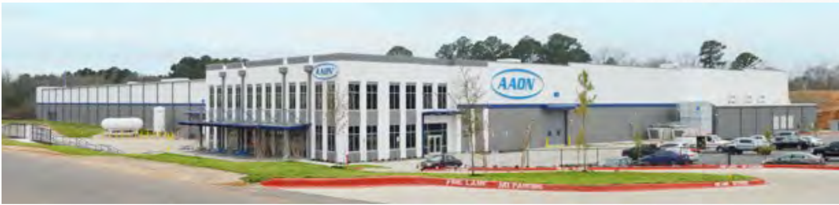
AAON Longview Expansion – Beginning Operation in 2021
