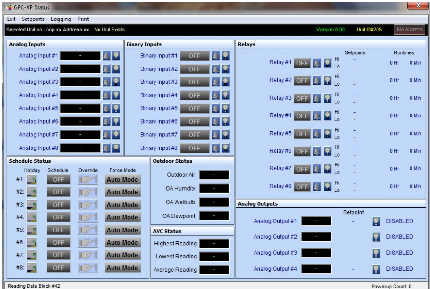
Figure 8: GPC-XP Controller Status Screen
