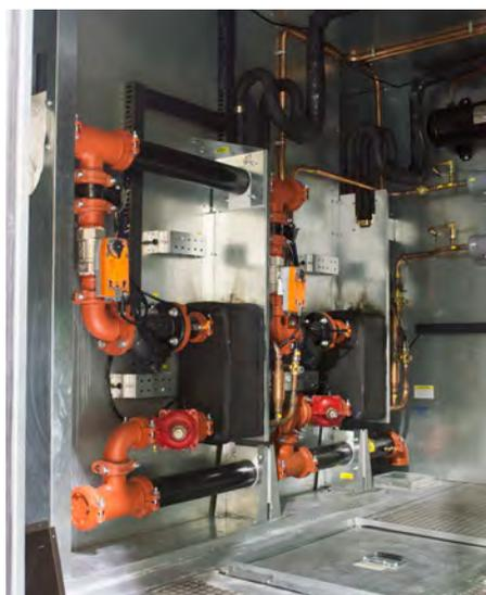
▲ Refrigerant-to-Water Heat Exchanger Walk-In Service
